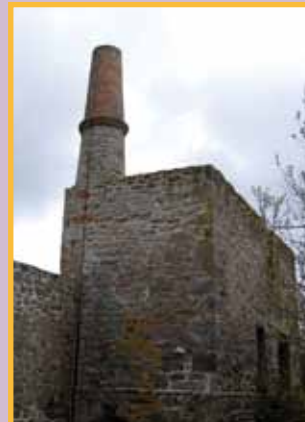
The 19th century engine house.
