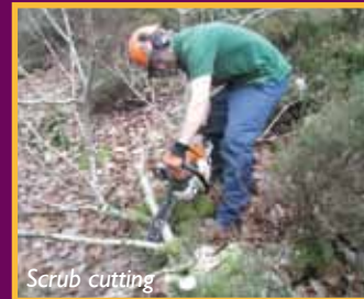
Cutting fire breaks
